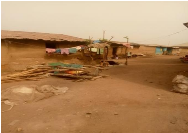
Figure 10. Derelict or slum settlements at Ago Area (Ijan-Odo Ado RDC, Ado-Ekiti) (Field Survey, 2023)
