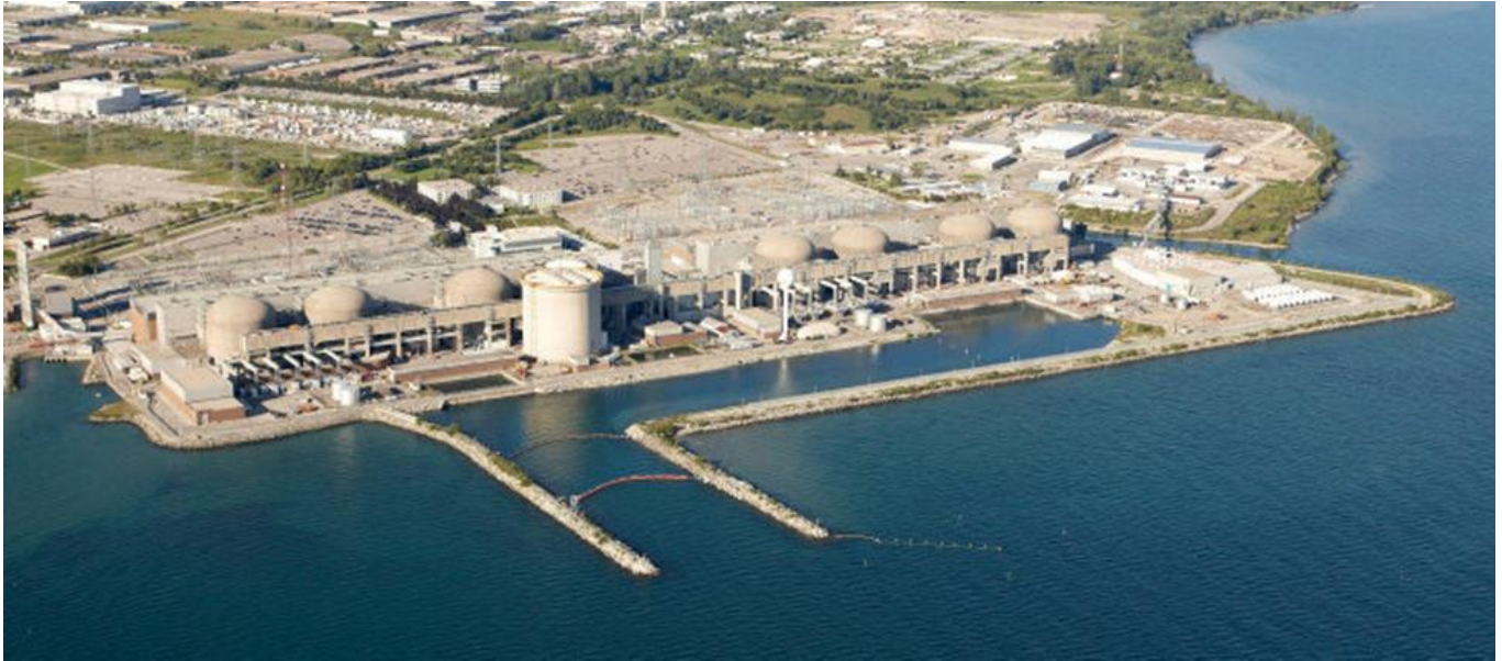
Figure 1. External view of the 3100 MW Pickering Nuclear Generating Station, showing its eight units, in Ontario, Canada. [Copyright © Ontario Power Generation Inc., all rights reserved. This information is subject to the general terms of use set out in Ontario Power Generation Inc.'s web site ( www.opg.com ).]
